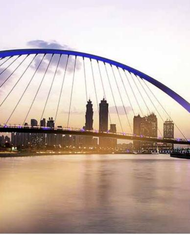
These bridges are what give the canal its unique look. Each bridge has a different structural form. There's a grand arch that's all curves, a low slung suspension bridge and a twisted truss. Although each of the bridges looks so very different, share steel as their main construction materials.
